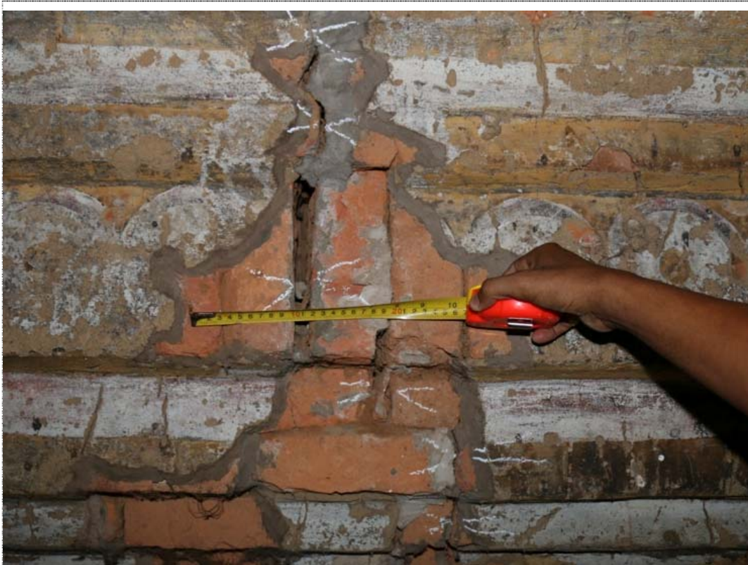
Fig. 42 The cracks were marked with chalk and then documented in detail with a scale bar in the photo to provide information about the width of the crack.
