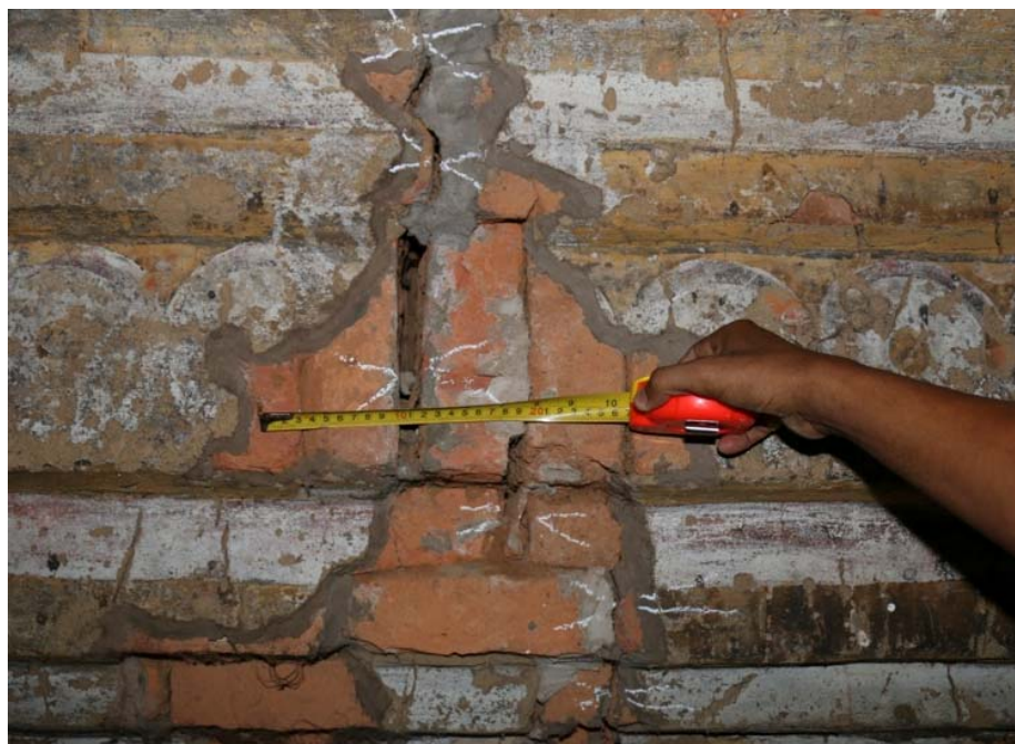
Fig. 7 First the cracks are marked with chalk and then documented in detail using a scale bar in the photo in order to provide information about the width of the crack.
