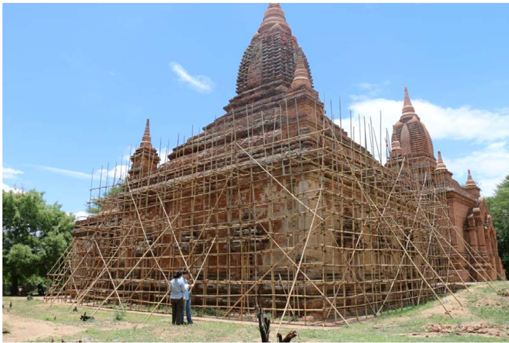
Fig. 3 A Bagan monument prepared for in-depth condition assessment. The access was secured and vegetation cleared in a radius of about 3-5 meters before setting up the scaffolding around building parts that need investigation.
