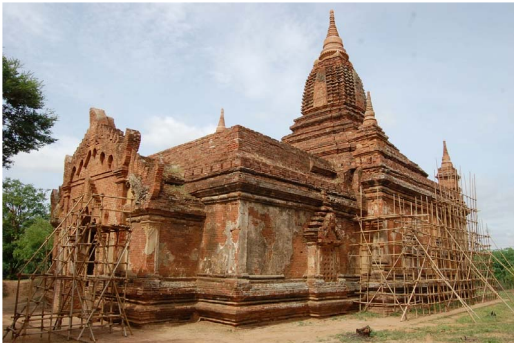
Fig. 35 Phaya-shwe-gu Temple with scaffolding installed for the areas that needed to be inspected, plus a moveable scaffold that can be used for accessing different parts of the exterior building.
